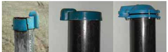
*Is your well head protected? The cracked wellhead cap on the left is an easy way to allow pollution into your well. Although the well cap in the middle looks better, it is a non-sanitary version. It provides better protection, but may leak. The sanitary cap on the right provides maximum protection at a slightly higher cost.*
